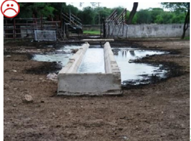
Leaking trough.
