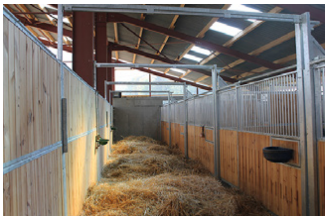
Sliding-partition system whereby the partitions between the stalls can be retracted to allow a tractor to pass through easily.
