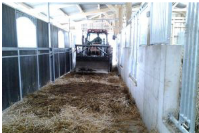
Sliding-partition system whereby the partitions between the stalls can be retracted to allow a tractor to pass through easily.
